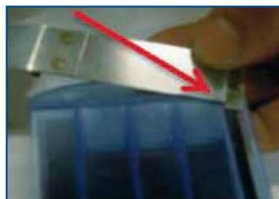
Place the end of the bracket 3 mm into the slat (the bracket is attached to the second slat from the end).
