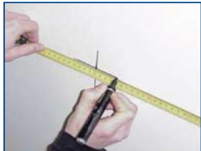
Mark the dimensions of the wall duct.
