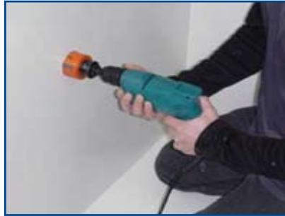
Drill the recess. Recess diameter:
