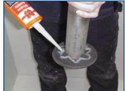
Apply sealant to gasket.
