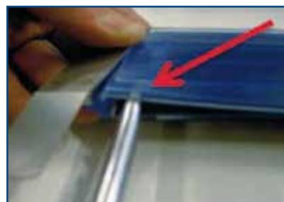
Open the groove of the slat with a screwdriver and slide the bracket over the slat.
