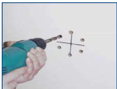
Remove bearing block and drill
