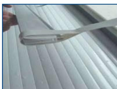
Slide the first slat through the straps with the spring towards the tube.
