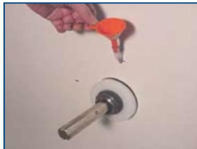
Fully insert funnel pouring hose into pouring channel.
