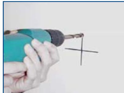
Drill first hole with Ø11 mm drill.
