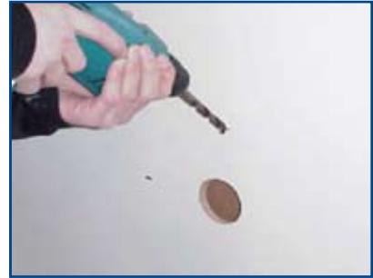
Drill a Ø12 mm pouring channel in the motor well at a 45° angle starting approximately 7 cm above the recess, through which the resin can be poured.
