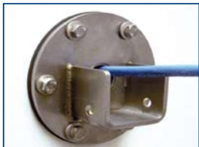
Carefully feed the cable of the tube motor through the hole.
