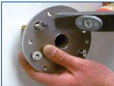
First thread the WAKO plugs onto the countersunk bolts, then position the pre-assembly flange and drive in the bolts until they are flush with the flange.
