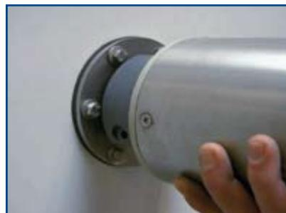
Slide the winding tube over the U-profile. ATTENTION! Continue to feed the cable through so it won't be damaged.
