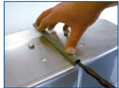
Install an electrical conduit through which the cable can pass under the edge tile (so the motor can be replaced in the future if necessary).
