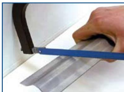
Saw the cable conduit to length, measured from the end with the mounting holes.
