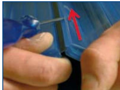
Place a thin, flat screwdriver between the hook and the groove and slide it toward the other end of the slat so the hook comes loose from the groove.
