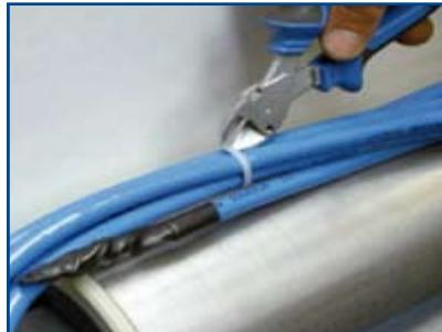
Cut the cable loose with wire cutters.
